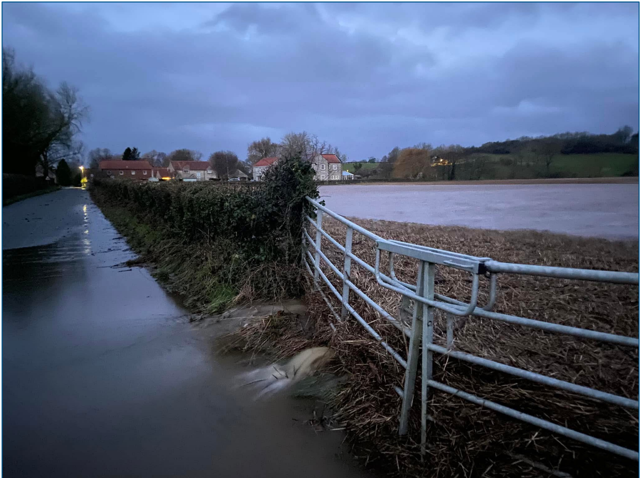
Figure 15 Photo of gate with vegetation blockage in Marton
